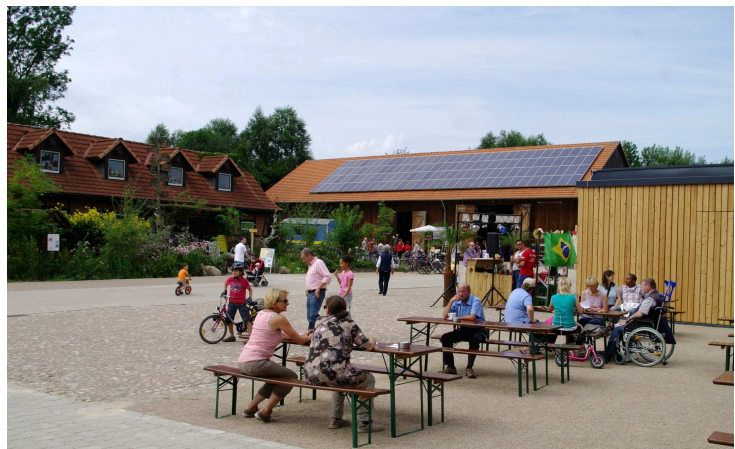
Gut Karlshöhe: Barn with photovoltaic system
