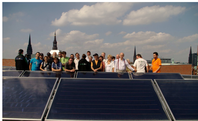
Solar thermal collectors in the Hafencity-Hamburg
